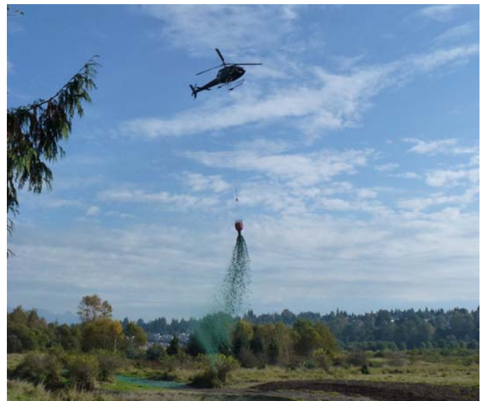
Photo: Using helicopter to spread the hydro-seed mixture and a 1,000 litre Bambi bucket
