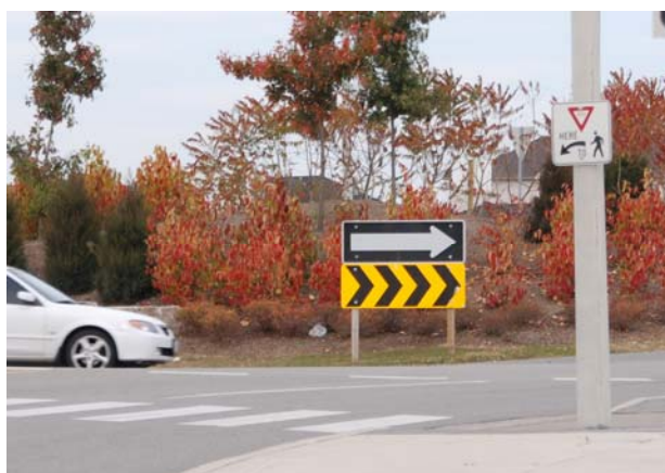
Figure 8.1 "Yield Here to Pedestrian" Sign at Pedestrian Crossing
